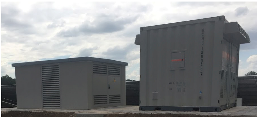
Figuur 10: Impressie transformator/inverterstation
