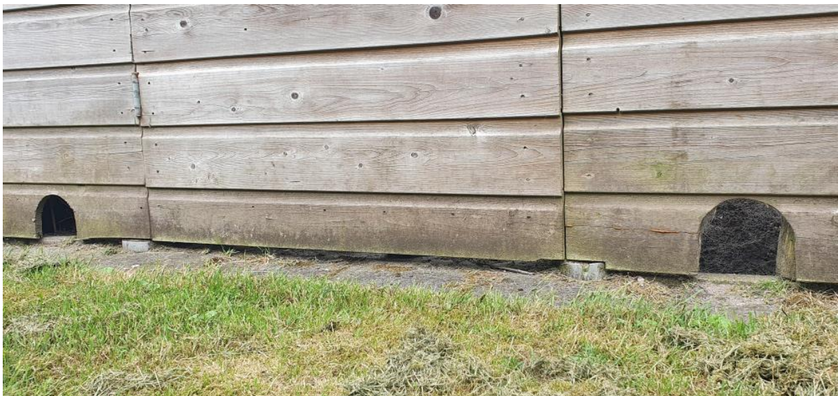
Figuur 17. Egelopening in schutting.
