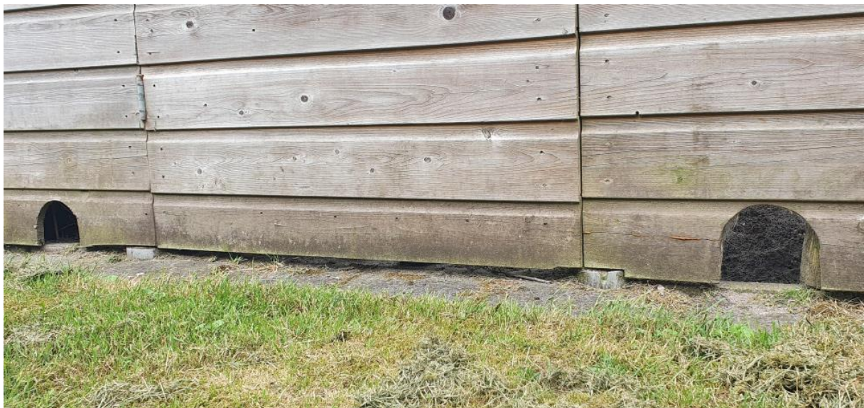
Figuur 17. Egelopening in schutting.
