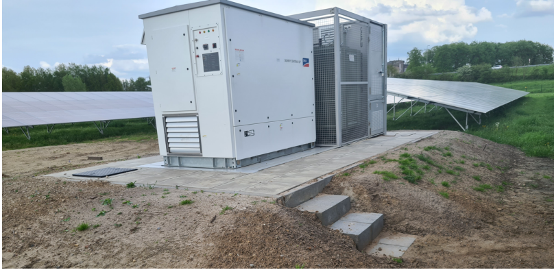
Figuur 10: Impressie transformator/inverterstation
