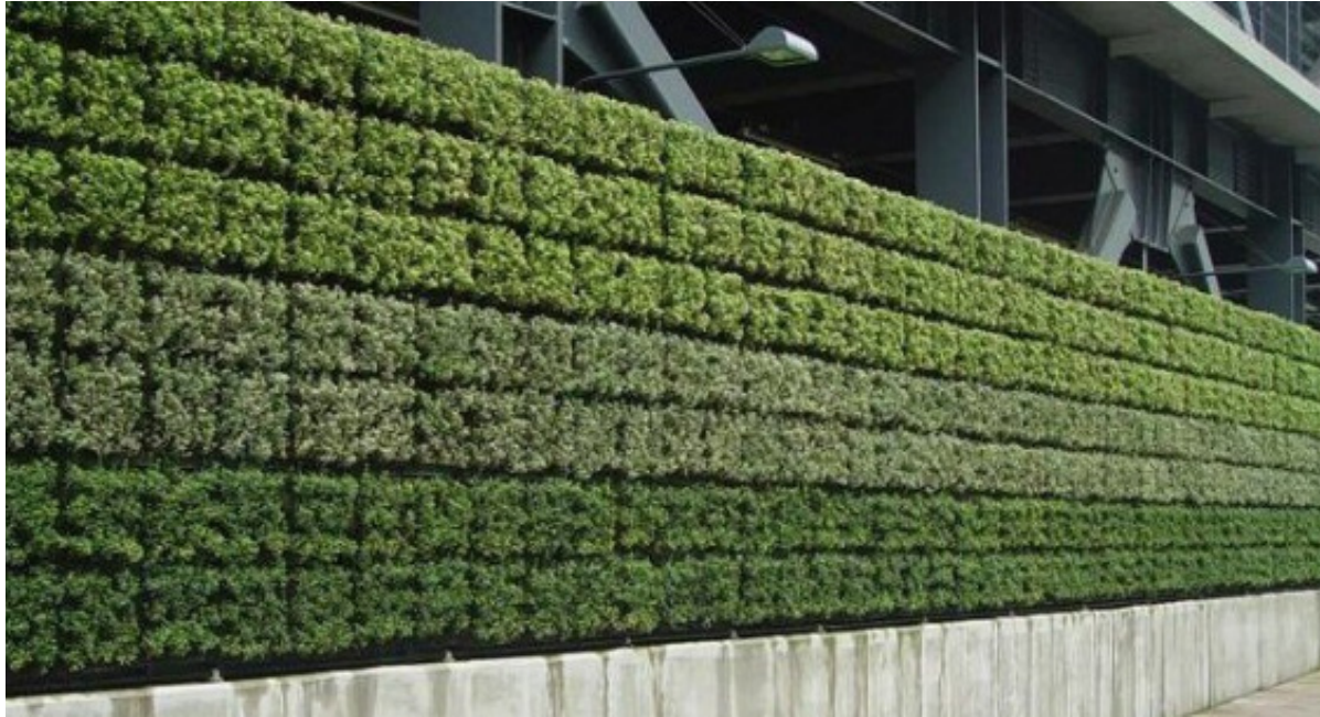
vertical green wall (van access irrigation)
